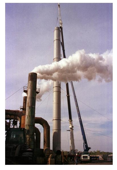
**Heil FRP Composite Stack** - A major lime producer ran afoul of neighbors and the state EPA when the discharge gas from their kilns drifted across adjoining properties. The existing stainless stacks were badly corroded and were not tall enough to meet EPA requirements. The solution was to replace the two stainless steel stacks with one FRP composite stack large enough to handle both discharge gas streams and tall enough to meet EPA requirements.
